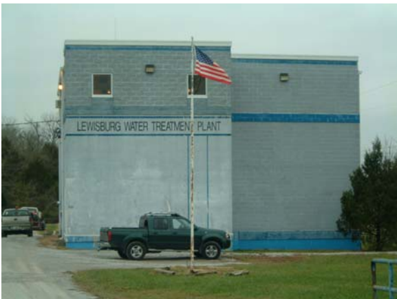
Lewisburg Water Treatment Plant (Lewisburg-Logan Co.)
